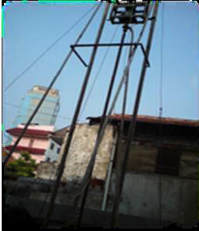
Gambar 2.32 Bored pile gawangan (Sumber: www.arsitur-pengertian-pondasi-bored-pile.com )
