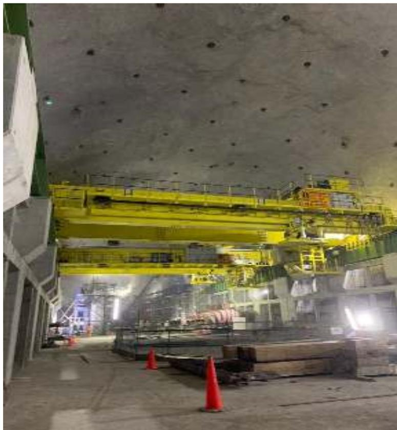
Gambar 3.3 *Underground Powerhouse*
