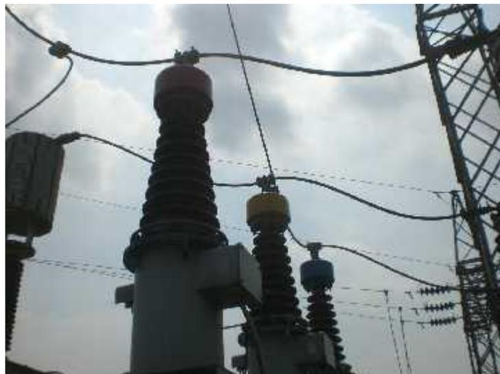
Gambar 3.3. Current Transformer G.I Pematang Siantar
