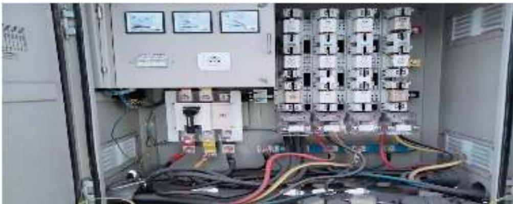
Gambar 3.9: Panel Transformator
