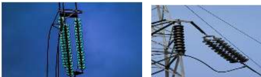
Gambar 2.6 insulator ceramic dan insulator kaca
