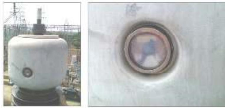
Gambar 2.15 Indikator Level Minyak Bushing
