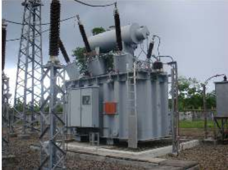
Gambar 2.15. Transformator Tenaga / Transformator Daya (TD)
