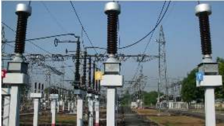
Gambar 2.13. Transformator Arus (CT)
