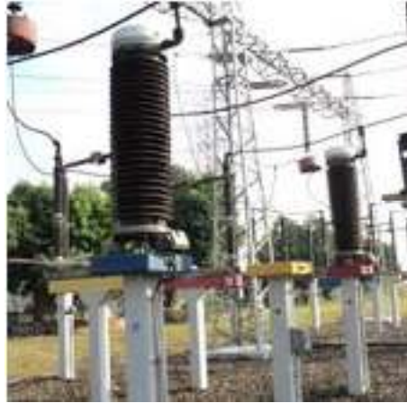
Gambar 2.11. Transformator Tegangan (Potensial Transformer)
