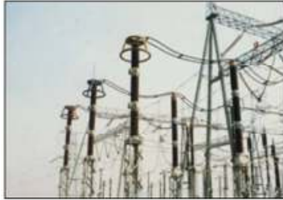
Gambar 2.10. Lightning Arrester (LA)
