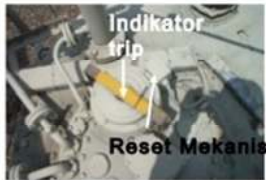
Gambar 2.4. Relai Tekanan Lebih (Sudden Pressure Relay)
