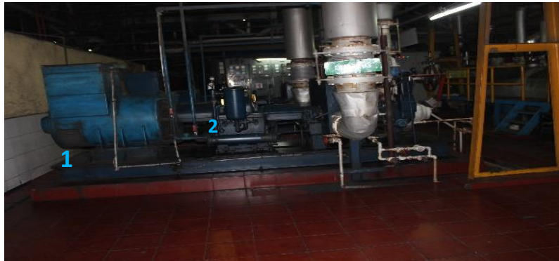
Figure 4.1 Variation of engine speed is measured at four points of measurement that is at 2 points on the steam turbine generator stand.
