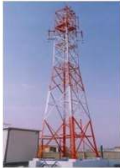
Gambar 2. 1 Tower BTS 4 Kaki (Rectangular) (Aslimeri, 2008)
