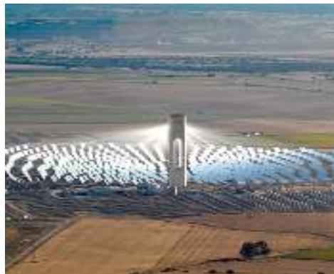
Gambar 2.12 Solar Power Plant
