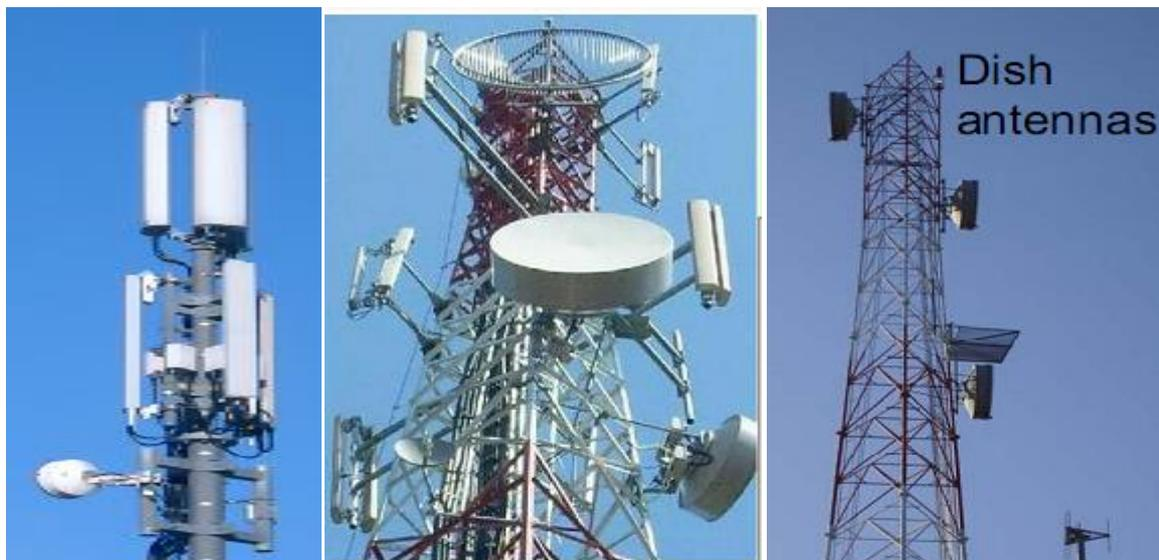
Gambar 1. Antena BTS
